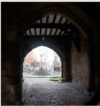
View through the Gatehouse to the Market Cross.
